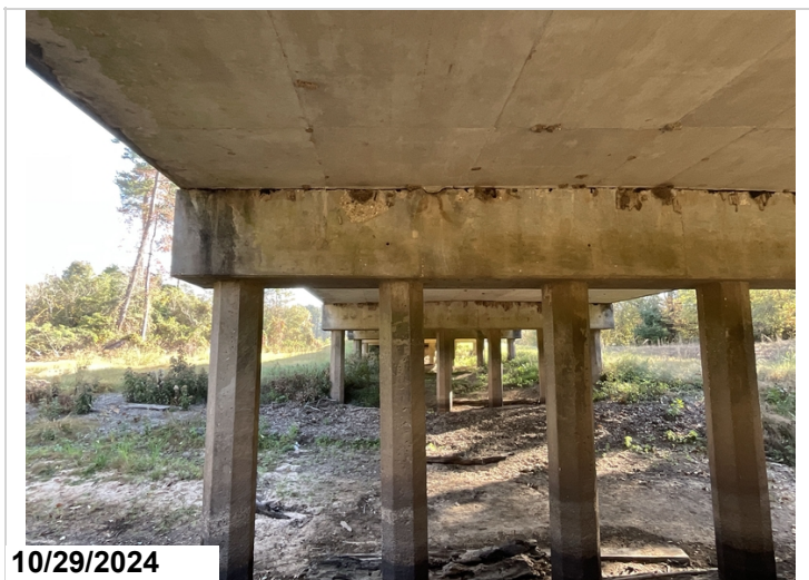
Bent 4, cap, back side above Pile 2, 2LF spall CS3
