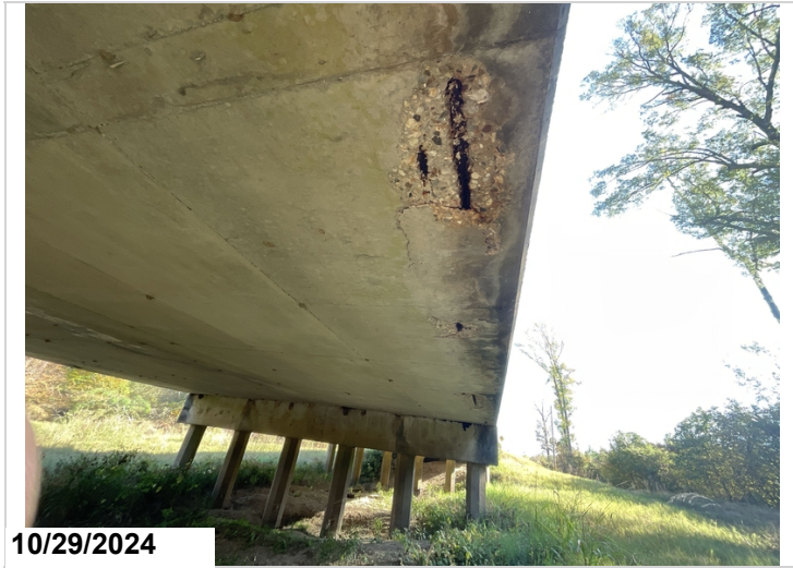
Span 5 under surface, right side, 12SF spall CS3.
