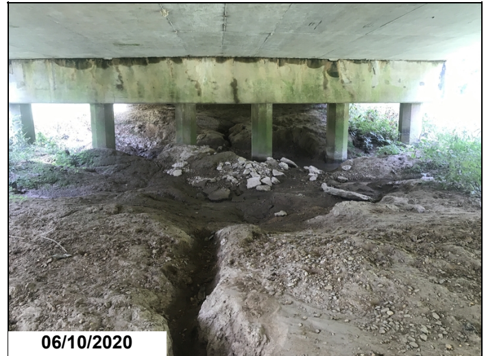
Bent 2 has minor erosion.
