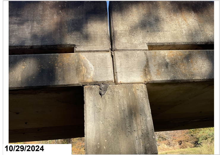
Span 4 & 5, right edge, at Bent 5. 1SF cracking CS2.
