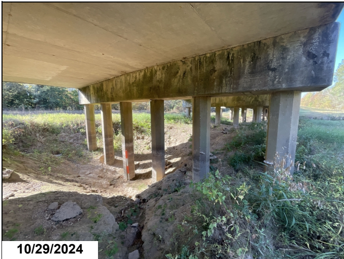
Bent 7, piles 3 - 6 have local scour 4' deep.
